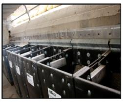
stormwater runoff for new or retrofitted sites by absorbing oil and grease and capturing trash and sediment, making it a truly comprehensive solution geared at removing key contaminants and pollutants from stormwater runoff. In addition, Smart Sponge<sup>®</sup> Plus incorporates an intrafilter antimicrobial to promote and prolong the effective and efficient functioning of the filter.
